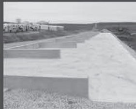
Reinforced Concrete Pad
