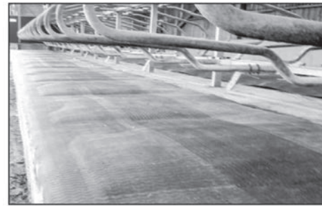
Renovation of the damaged mattresses with Aquatop
